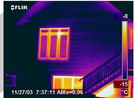
Thermal image of a Logix Home showing minimal heat loss
